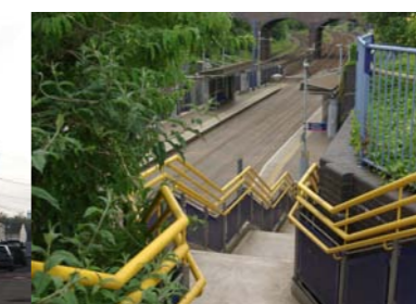
Hawthorns Metro station
